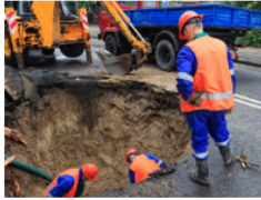
August 2020: Utilities and Public Rights-of-Way
